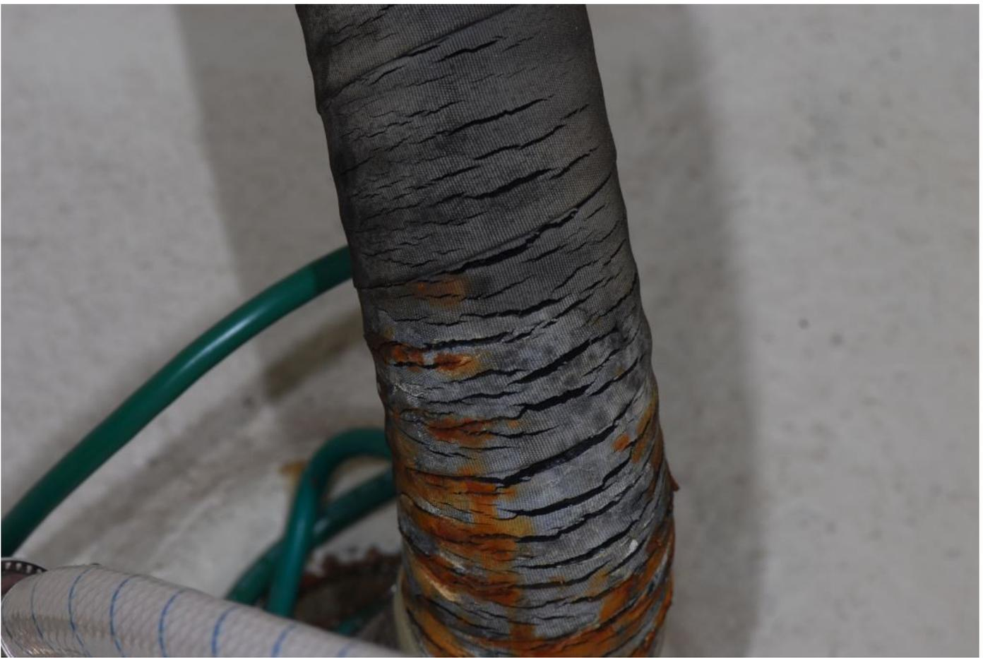
**Nearly all flooding that is the result of failed below the waterline plumbing is preventable. Inspect your raw water systems regularly.**
